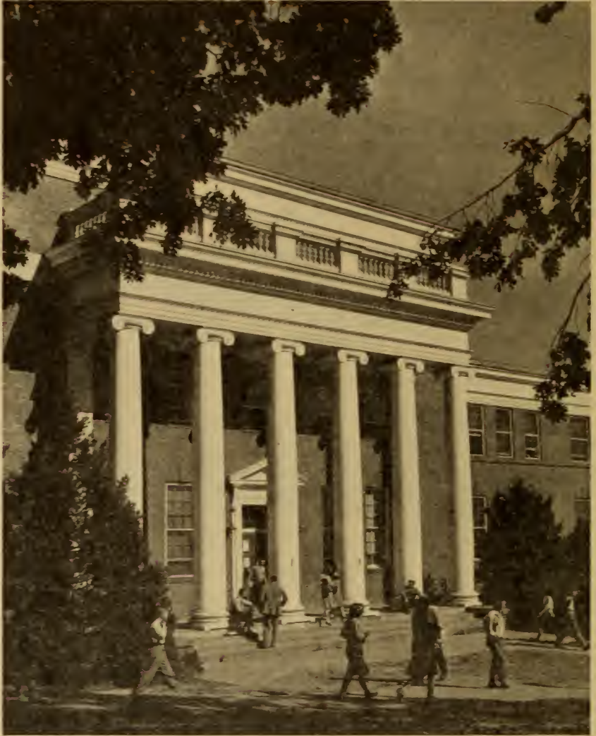
Campus Building, University of Maryland College Park, Maryland
